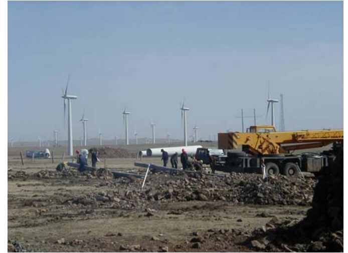
Wind farm under-construction
